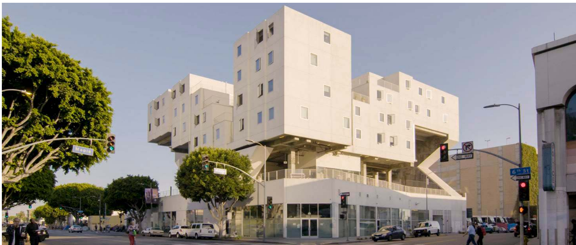
Star Apartments, Los Angeles
